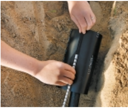
2 Sleeve is positioned over splice or damaged area and closed with metal channel.
