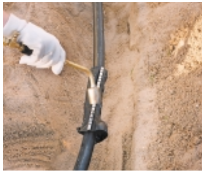
3 Heat is applied to shrink the sleeve and melt the adhesive liner.
